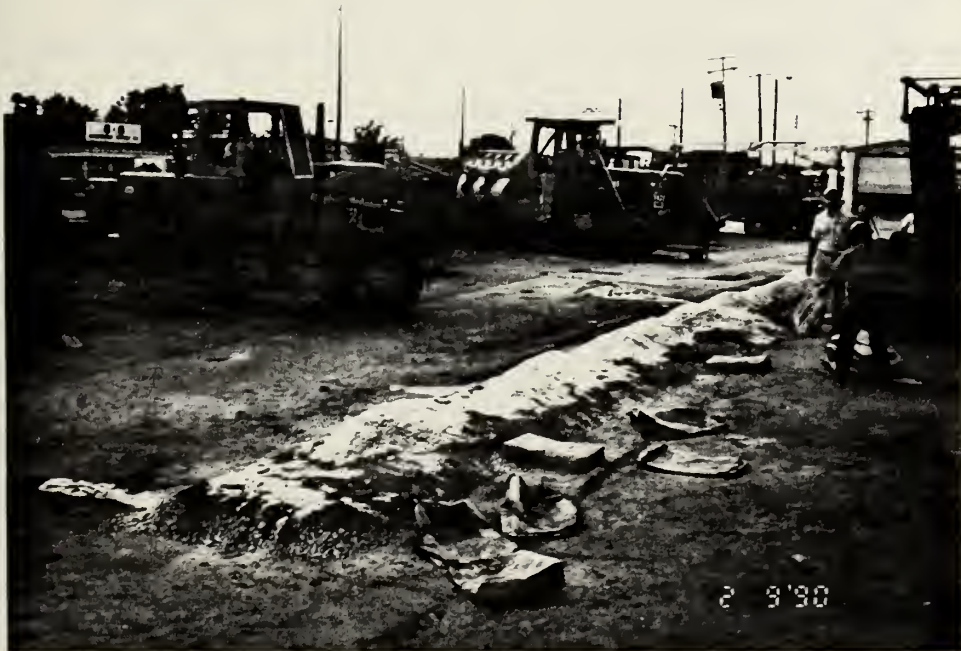
Figure 2.8 Cement Powder Placement With Sand Cover
